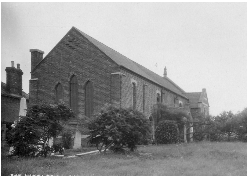
Photograph of the rear of the Chapel after reconstruction of new rear elevation to the same height as the frontal part in 1920s. The new housing for the organ can also be seen.
